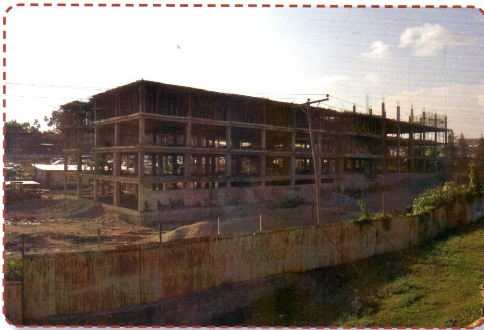
Special Department Stores & Recreation Centre (Under Construction) - Akaki -Kality
