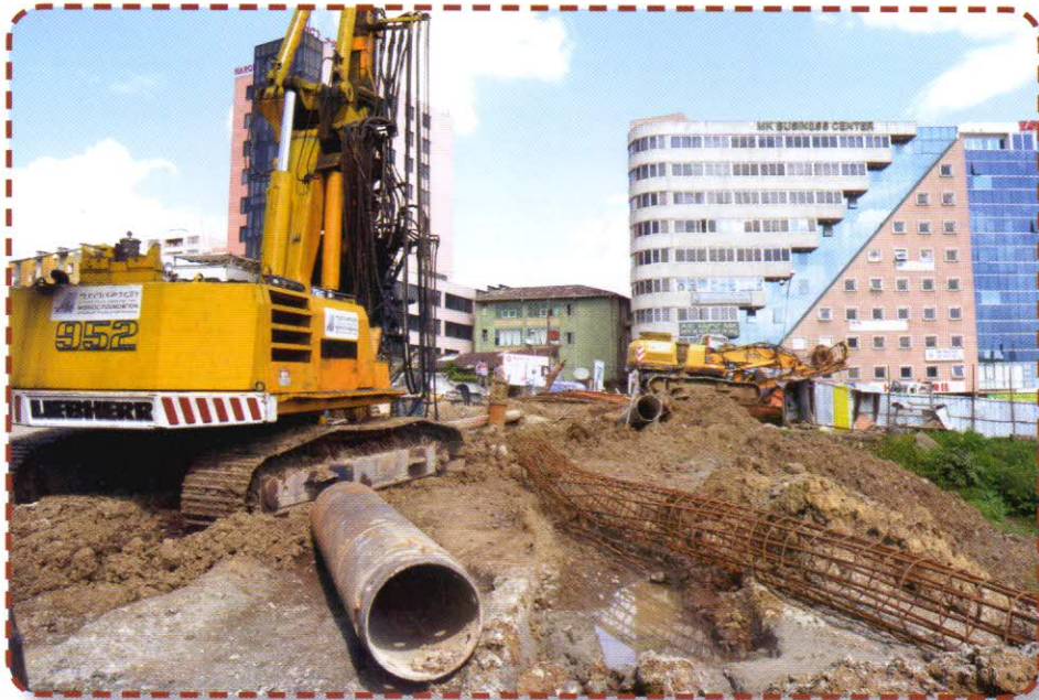
Future Head Quarters (Under Construction) - Tewodros Square
